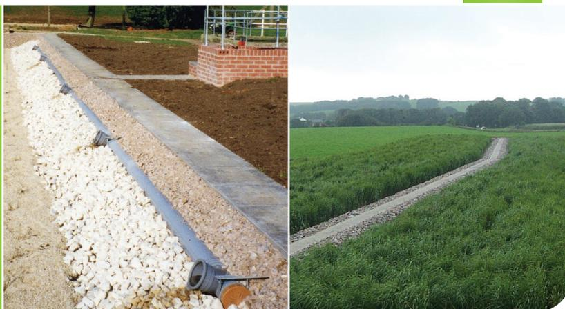
**H**orizontal Flow (HF) reed beds consist of an excavation approximately 0.6 metre deep which is lined to ensure untreated effluent cannot percolate down into the groundwater. The bulk of the excavation is filled with single sized media such as gravel with larger media at the inlet and outlet. A piped inlet distribution and drainage system is installed and reeds are planted directly into the gravel media. The effluent to be treated passes through the gravel media and the level
