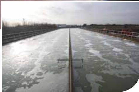
ARM reengineered the distribution and collection system and retrofitted FBA™ into the existing reed beds. The open water zones were filled with gravel and the gravel depth increased by 500mm. The upgrade works at the Mayfield Farm included the addition/modification of:
