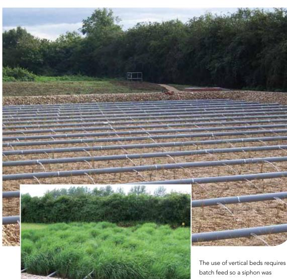
batch feed so a siphon was installed to negate the need for batch pumping and power connection. Two beds of 20 m x 40 m were constructed totalling 1,600 m<sup>2</sup>. A stilling chamber
