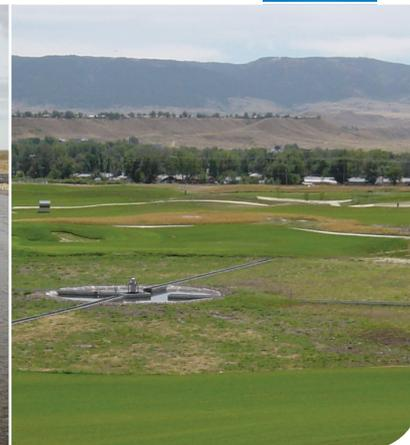
**F**orced Bed Aeration™ (FBA™) is a new wastewater treatment technology which enhances constructed wetland treatment performance. Significantly higher contaminant removal rates are attained along with an increased consistency of performance. Developed in the USA, by our partners Naturally Wallace, FBA™ can be used in both horizontal and vertical flow constructed wetland systems. Blowing air through the wetland system
