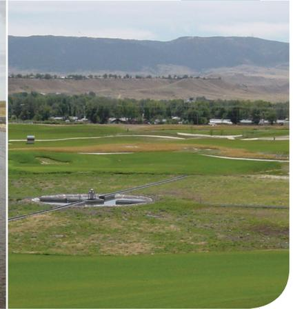
**F**orced Bed Aeration™ (FBA™) is a new wastewater treatment technology which enhances constructed wetland treatment performance. Significantly higher contaminant removal rates are attained along with an increased consistency of performance. Developed in the USA, by our partners Naturally Wallace, FBA™ can be used in both horizontal and vertical flow constructed wetland systems. Blowing air through the wetland system
